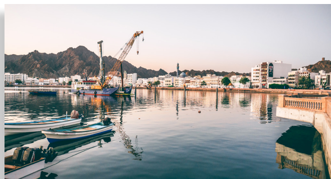
Sultan Qaboos Port, which is being repurposed as a $2 billion waterfront destination.
